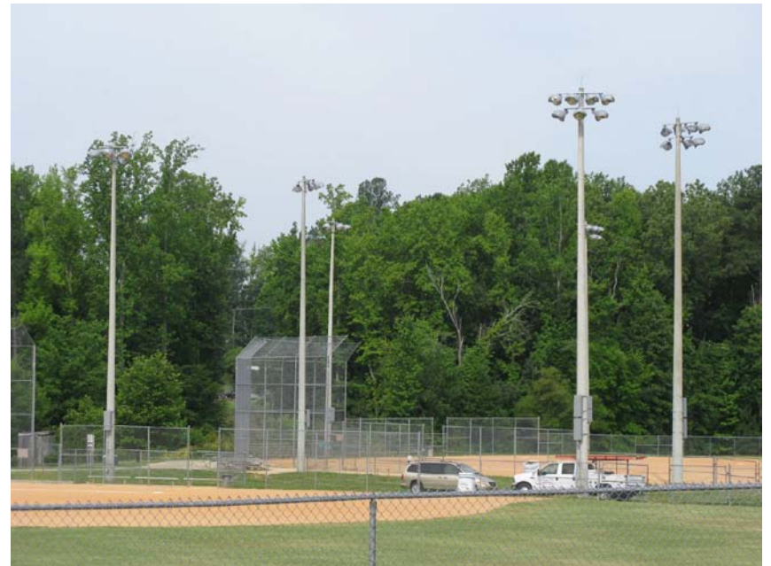
Softball Field Lights at Homestead Park
